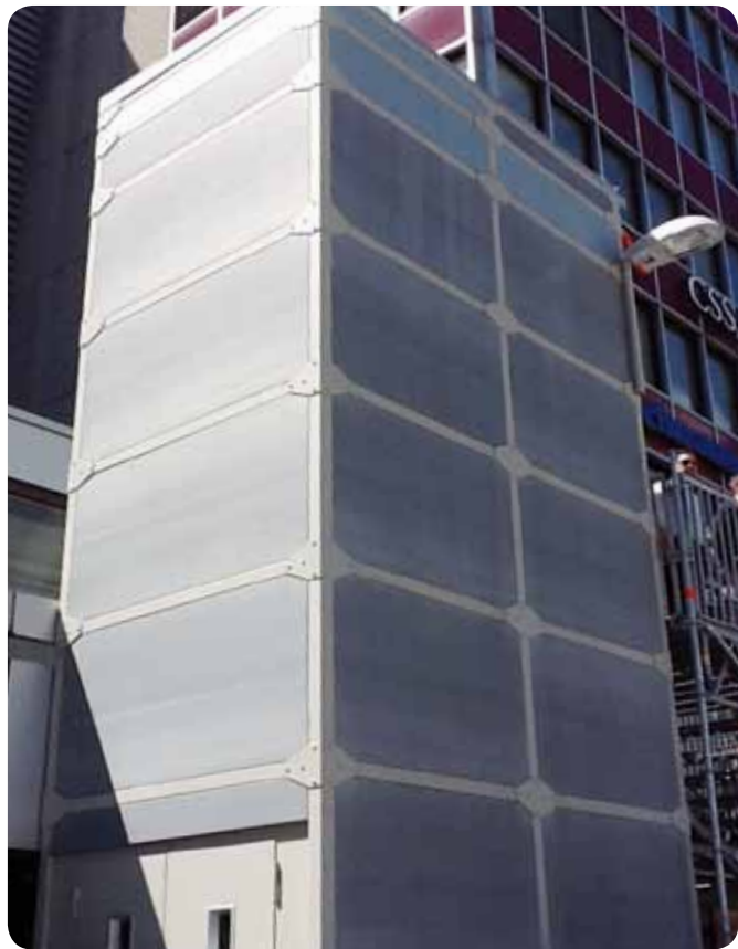
Construction-site lift sheet metal panels of galvanised sheet, frame struts primed
