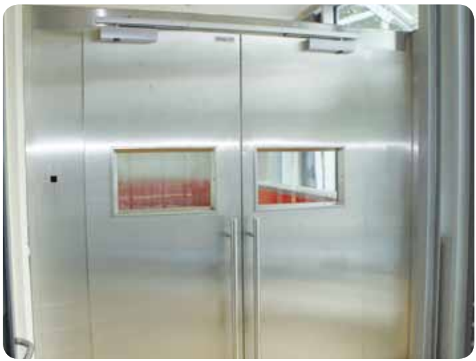
Two-wing door of V2A/304: internal hinges, rectangular windows, bar handles, with fire-protection closers (with control of closing sequence)
