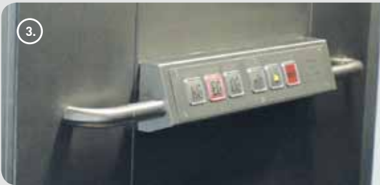
1. MRLH with automatic cabin doors 2. MRLH interior view of cabin 3. MRLH control unit as disability-friendly console in handrail
